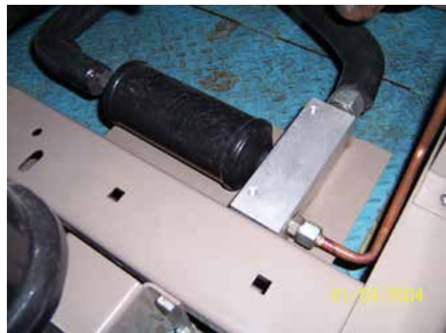
FIGURE 16 - EDUCTOR FILTER DRIER
