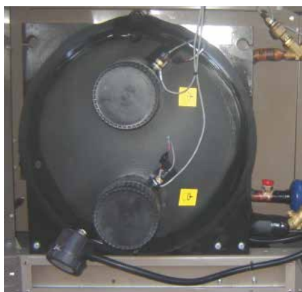
FIGURE 7 - 2-PASS EVAPORATOR WITH OPTIONAL IMMERSION HEATER
