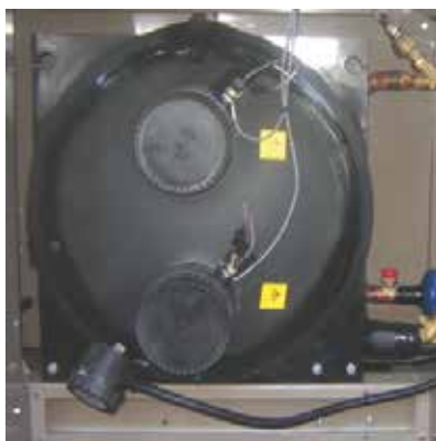
FIGURE 7 - 2-PASS EVAPORATOR WITH OPTIONAL IMMERSION HEATER
