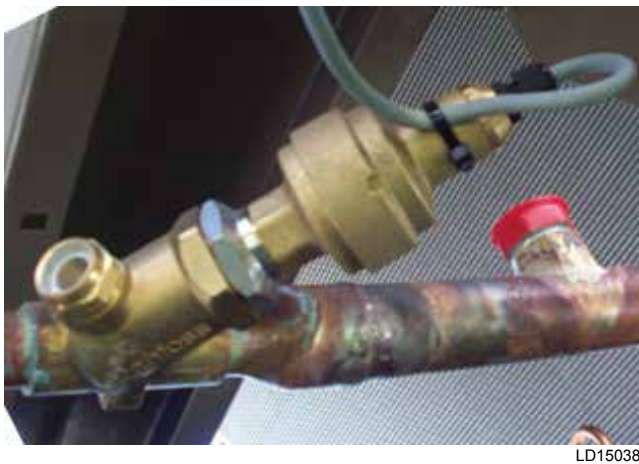
FIGURE 19 - ECONOMIZER STEPPER CONTROL VALVE
