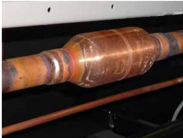
FIGURE 20 - CHECK VALVE
