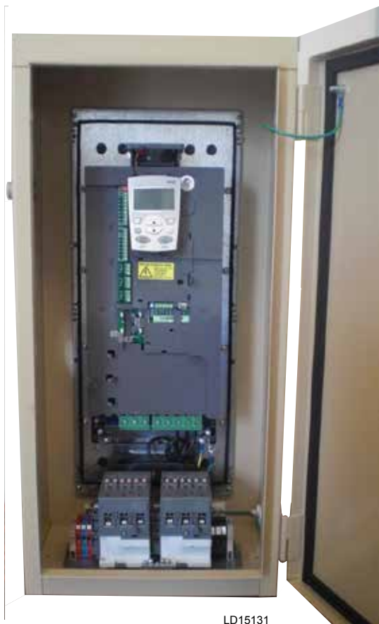
FIGURE 101 - INVERTER WITH KEYPAD AND DISPLAY INSTALLED
