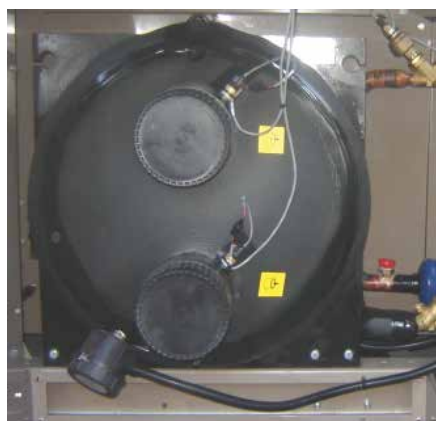
FIGURE 7 - 2-PASS EVAPORATOR WITH OPTIONAL IMMERSION HEATER
