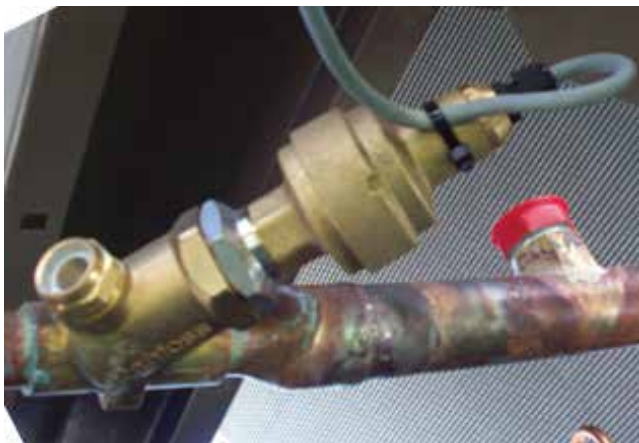
FIGURE 19 - ECONOMIZER STEPPER CONTROL VALVE
