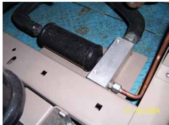
FIGURE 16 - EDUCTOR FILTER DRIER
