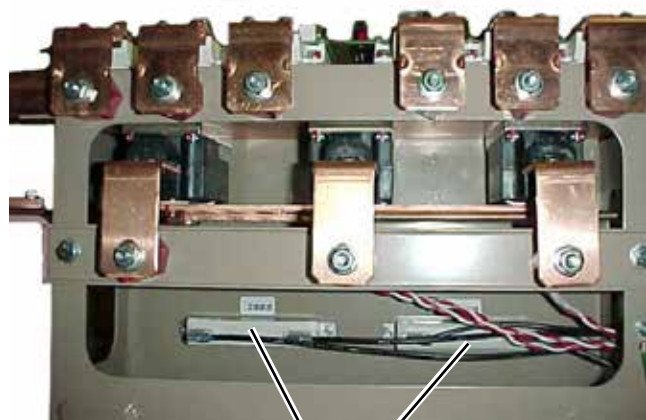
EQUALIZING/BLEEDER RESISTORS
