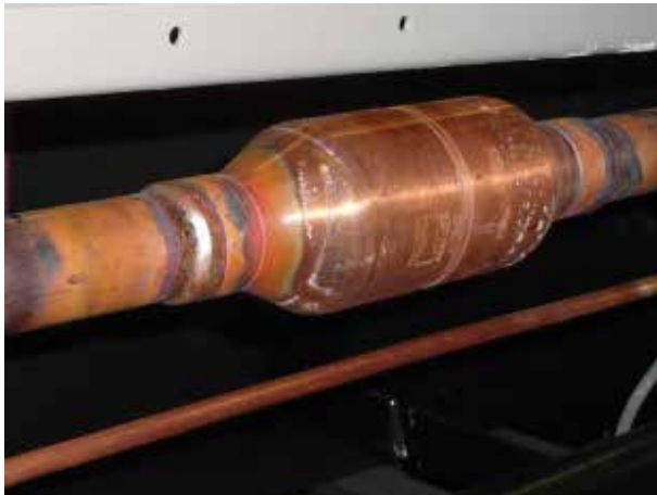
FIGURE 20 - CHECK VALVE
