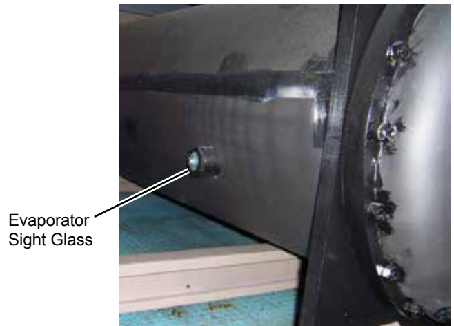
FIGURE 8 - EVAPORATOR SIGHT GLASS
