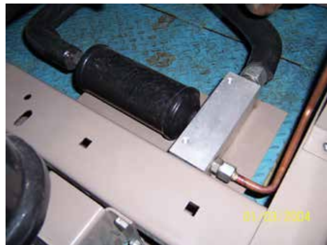
FIGURE 16 - EDUCTOR FILTER DRIER
