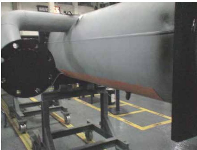
FIGURE 11 - SUCTION PIPING
