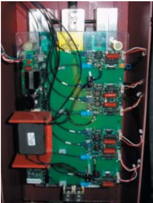
FIG. 11 – SCR POWER STACK ASSEMBLIES
