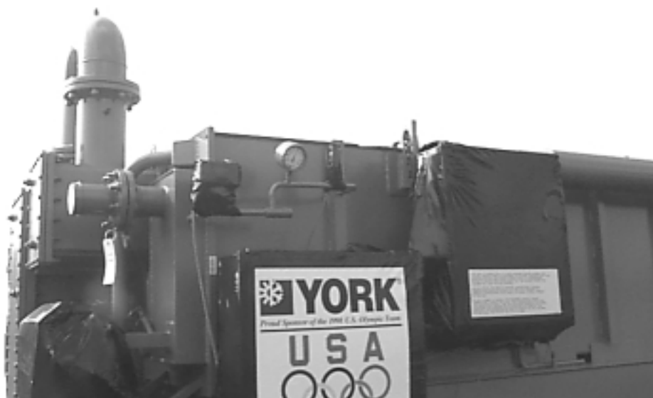
FIG. 2 – LOCATION OF PRESSURE GAUGE ON S-MODEL UNIT
