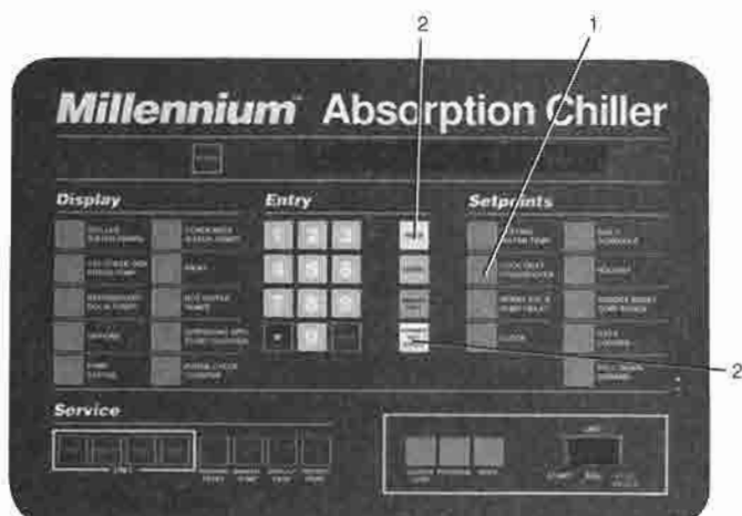
FIG. 6 - KEYPAD - PROGRAMMING "COOL/HEAT CHANGEOVER" SETPOINT
