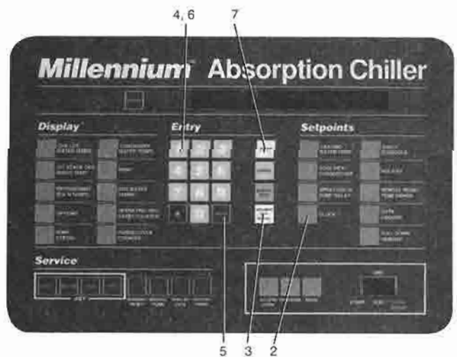
FIG. 7 - KEYPAD - PROGRAMMING "CLOCK" SETPOINT
