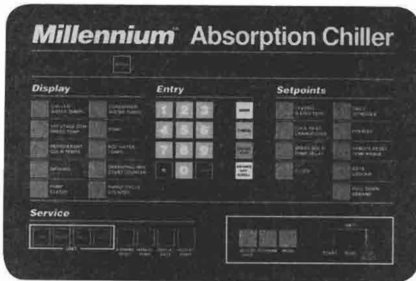
FIG. 1 - MICROCOMPUTER CONTROL CENTER AND KEYPAD
