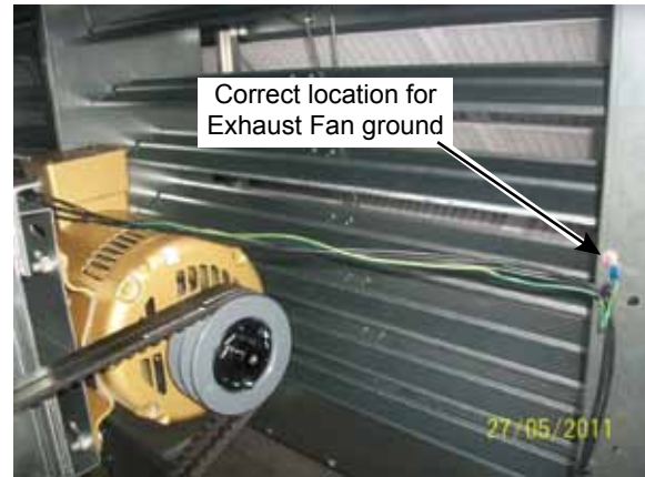
FIGURE 2 - CORRECT EXHAUST FAN GROUNDING
