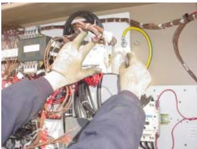
FIG. 8 - MARKING SMART RELAY BRACKET HOLE LOCATIONS
