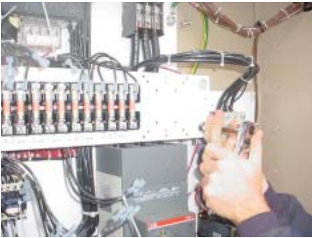
FIG. 3 - REMOVE FOUR SCREWS SECURING FUSE PANEL
