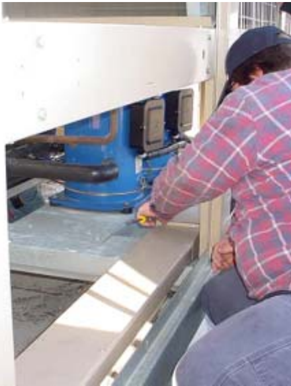
FIG. 16 - REMOVING WIRE RACEWAY COVER
