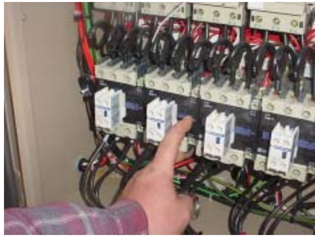
FIG. 14 - ENSURE CONTACTOR/TOP MOUNT AUXILIARY CONTACTS FUNCTION
