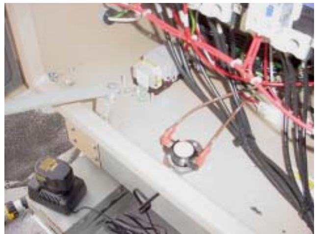
FIG. 24 - INSTALLATION OF OUTDOOR THERMOSTAT
