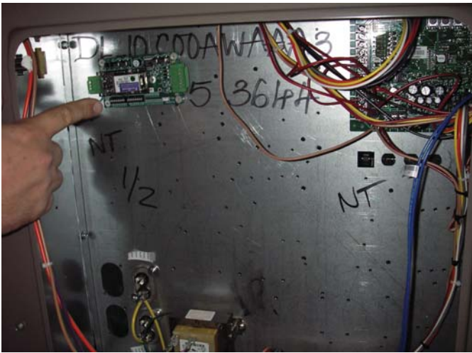
FIGURE 3: Simplicity®LINC Location in 6.5-12.5 Ton RTU
