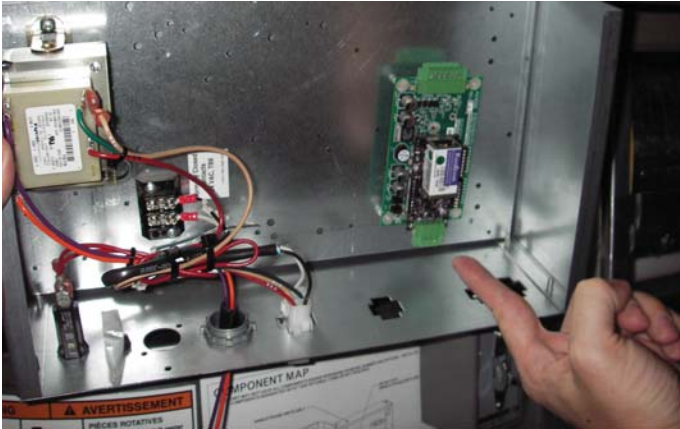
FIGURE 2: Simplicity®LINC Location in 3-6 Ton RTU, Wrapper for Intelli-Comfort™ Controls
