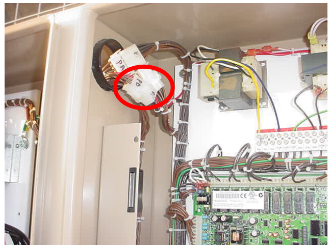
FIG. 11 - LOCATION OF PB/JB CONNECTION
