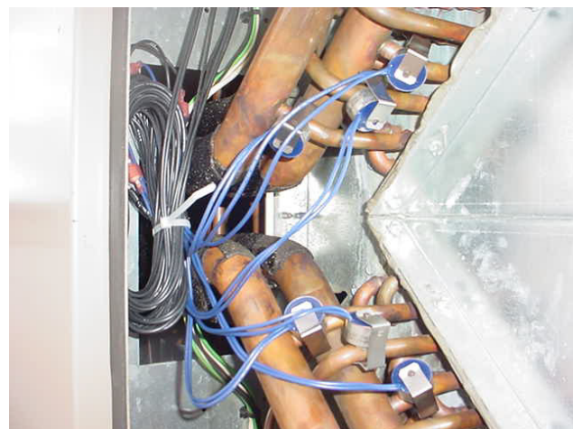
FIG. 23 - FINAL FREEZESTAT WIRING (6-COMPRESSOR UNIT SHOWN)
