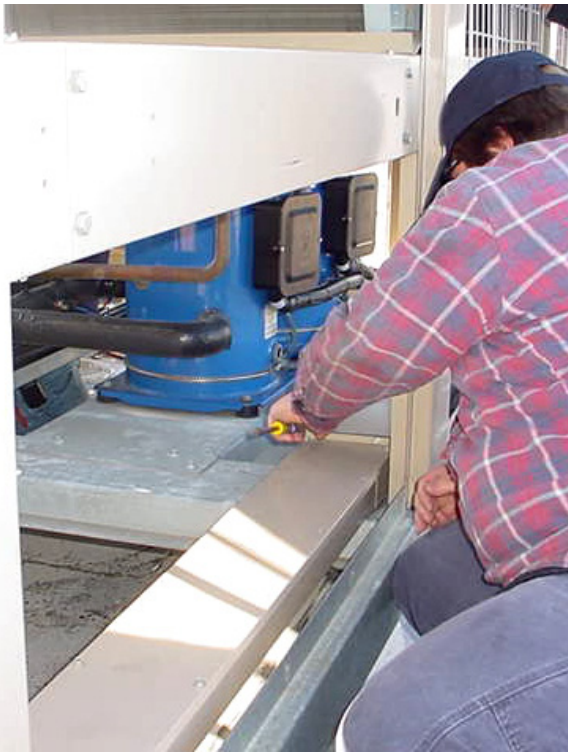
FIG. 16 - REMOVING WIRE RACEWAY COVER
