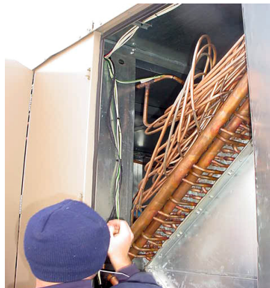
FIG. 18 - ROUTING FREEZESTAT WIRING FROM CONTROL PANEL TO COIL HEADER
