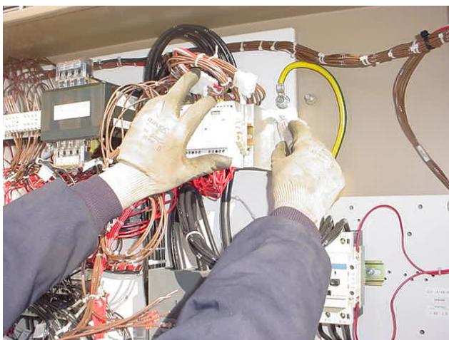
FIG. 8 - MARKING SMART RELAY BRACKET HOLE LOCATIONS
