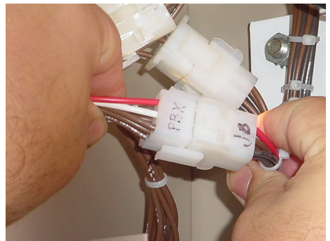
FIG. 12 - CONNECTING SMART RELAY HARNESS
