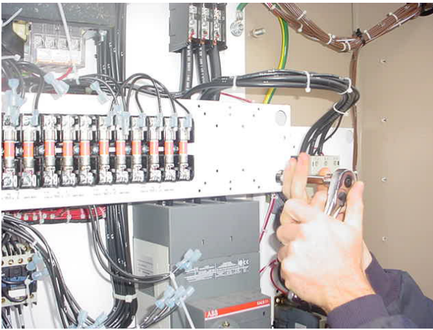
FIG. 3 - REMOVE FOUR SCREWS SECURING FUSE PANEL
