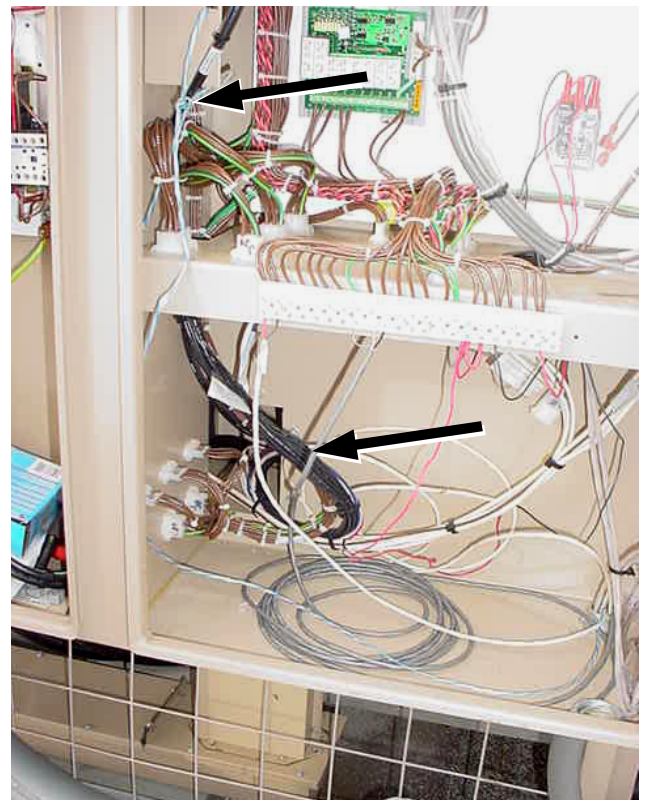
FIG. 17 - FREEZESTAT HARNESS
