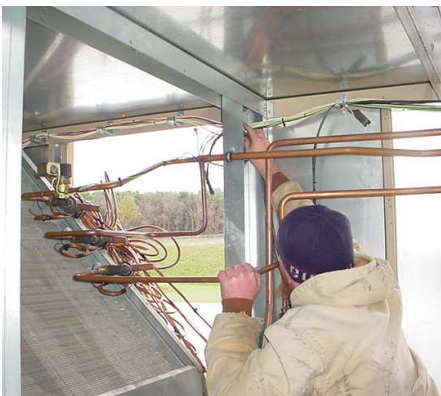
FIG. 18 - ROUTING FREEZESTAT WIRING FROM CONTROL PANEL TO COIL HEADER
