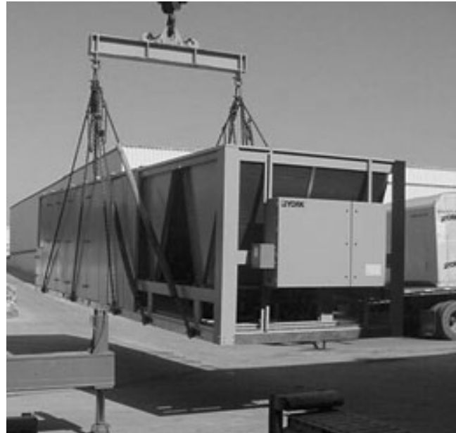
FIG. 2 – UNIT RIGGING
