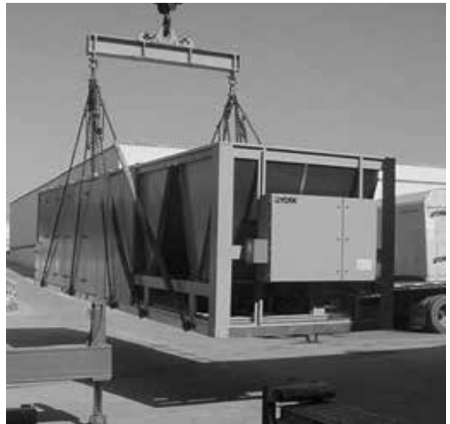
FIGURE 3 - UNIT RIGGING
