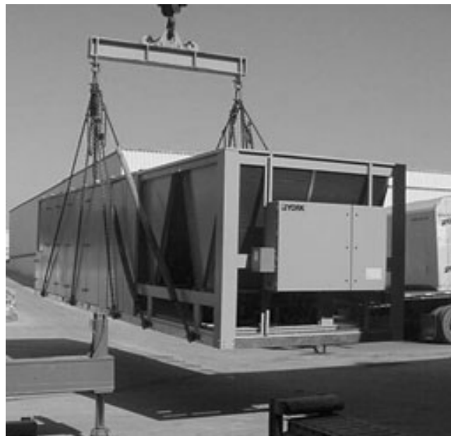
FIG. 2 – UNIT RIGGING
