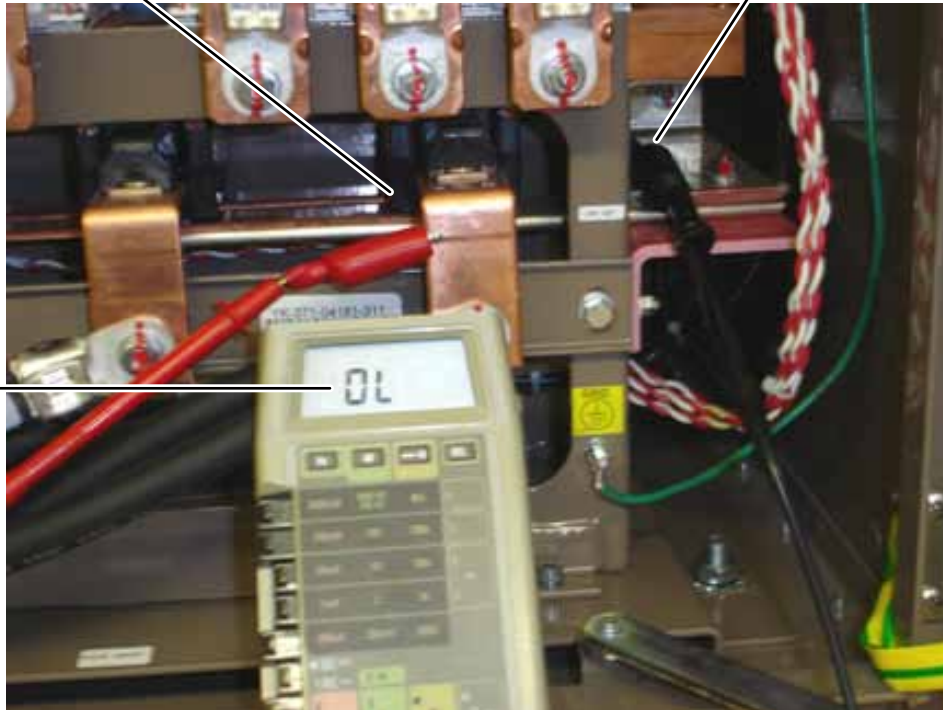
FIGURE 12 - SCR / DIODE MODULE VERIFICATION (REFERENCE STEP 1)
