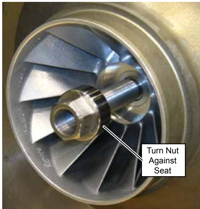
FIGURE 75 - IMPELLER MOUNTING NUT
