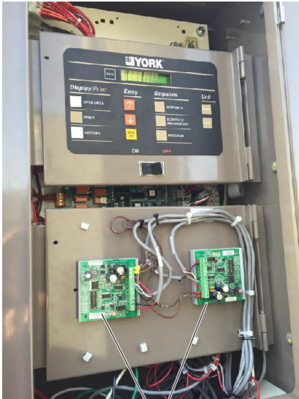
MOUNTING LOCATION OF THE SPORLAN (PARKER) CONTROLLERS
