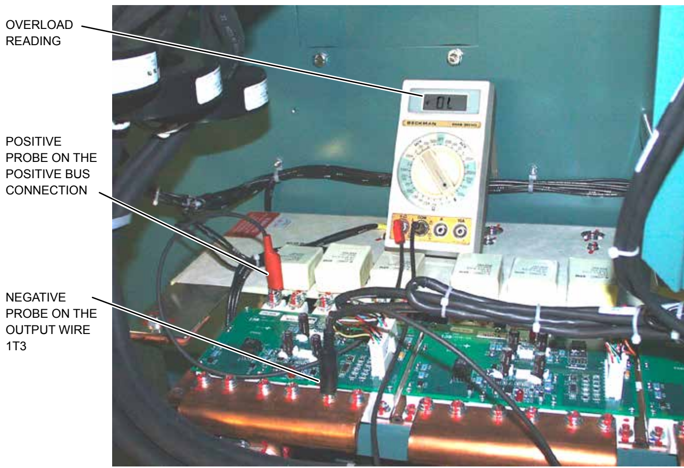
FIGURE 44 - 385/419/503/608/658/704/900 HP DRIVE IGBT MODULE VERIFICATION #1
