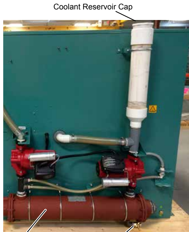
FIGURE 20 - COOLANT DRAIN CONNECTION INSIDE OF VSD
