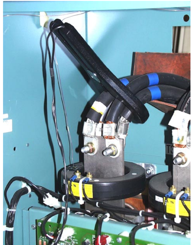
Figure 2 above shows the location of a current clamp-on. Ensure that the clamp-on is completely closed around the motor wire. Repeat this measurement for the other 2 phases.
