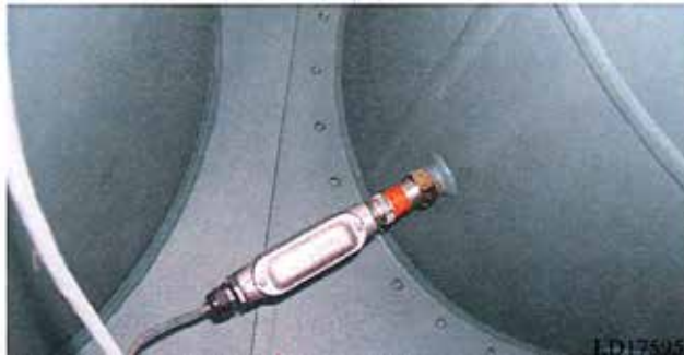
FIGURE 1 - REFRIGERANT LEVEL SENSOR
