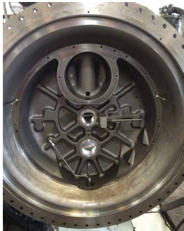
FIGURE 32 - BEARING HOUSING REMOVED
