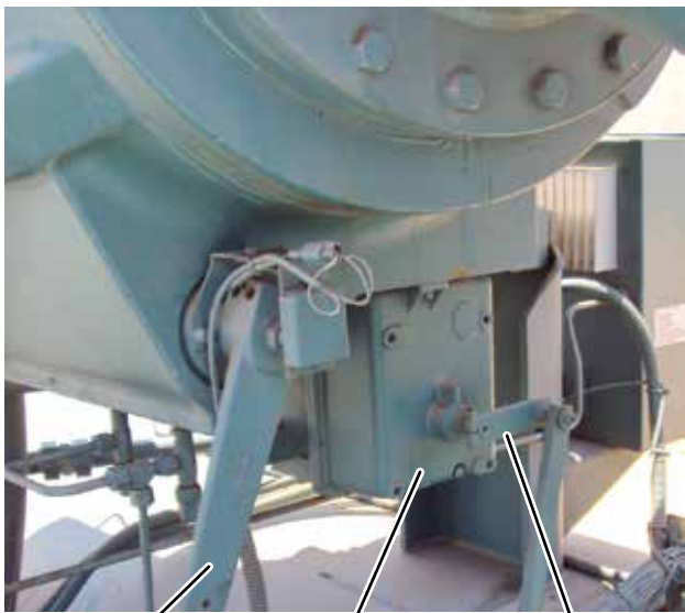
External Lever Vane Motor DETAIL A Linkage
