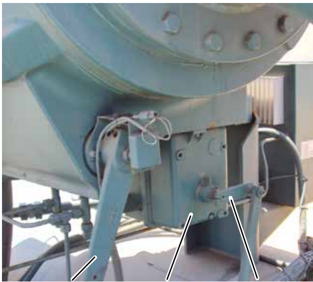
External Lever Vane Motor Linkage DETAIL A
