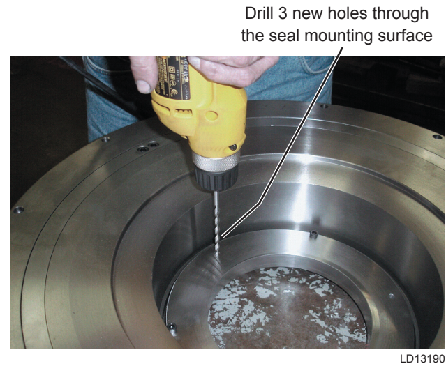
FIG. 4 - DRILLING NEW HOLES
