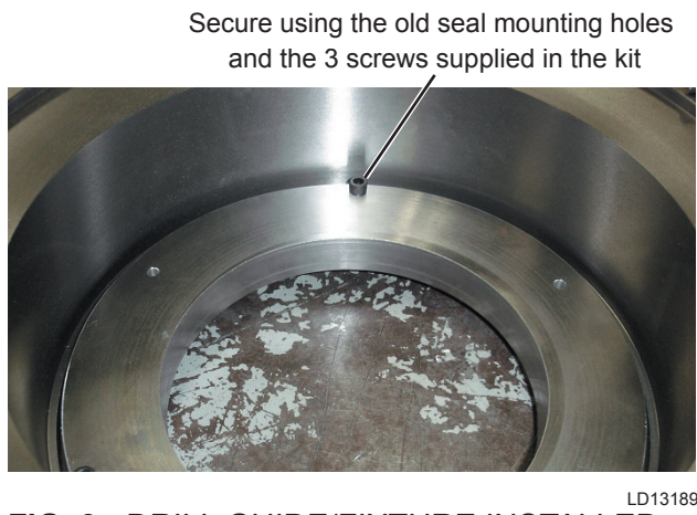
FIG. 3 - DRILL GUIDE/FIXTURE INSTALLED
