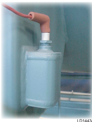
FIG. 1 – REFRIGERANT FLOAT SWITCH (1F)
