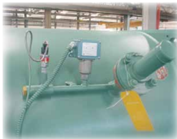
FIGURE 15 - RUPTURE DISK FROM FACTORY
