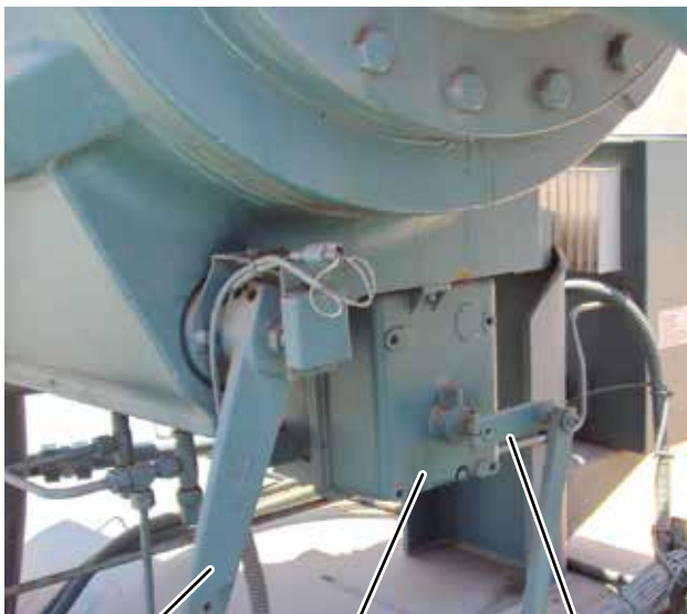
External Lever Vane Motor DETAIL A Linkage
