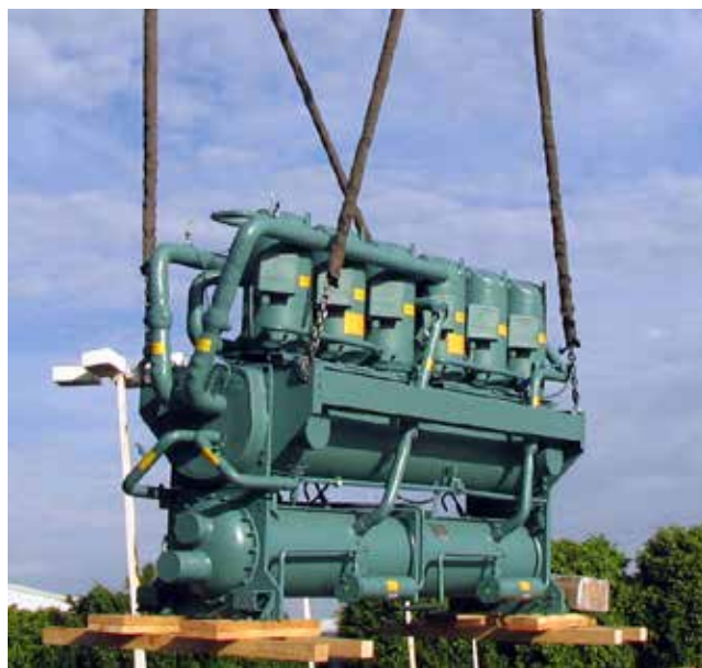
FIGURE 8 - CHILLER RIGGING AND LIFTING WEIGHTS
