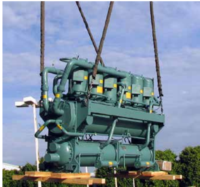
FIGURE 8 - CHILLER RIGGING AND LIFTING WEIGHTS
