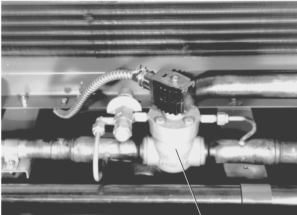
HOT GAS BY-PASS (OPTIONAL) SYSTEM #1
