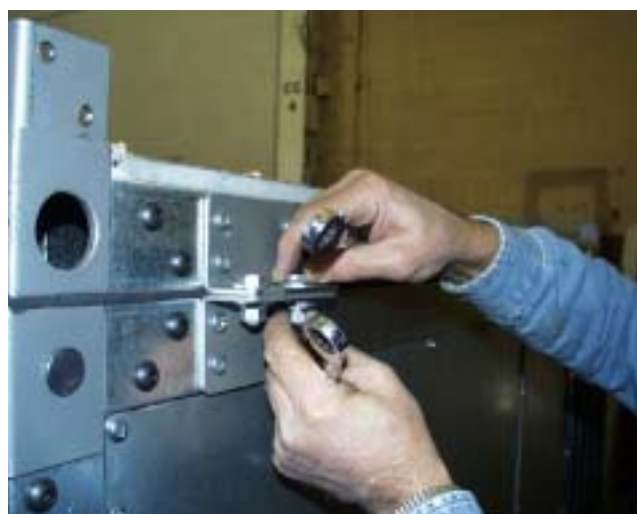
FIG. 11 - REMOVE HARDWARE FROM TOP SECTION MOUNTING BRACKETS
