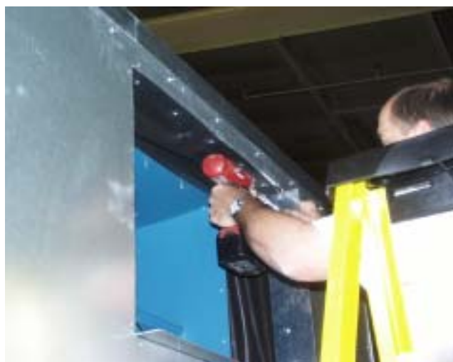
FIG. 4 - DISCONNECT FAN DISCHARGE FLEX CONNECTOR
