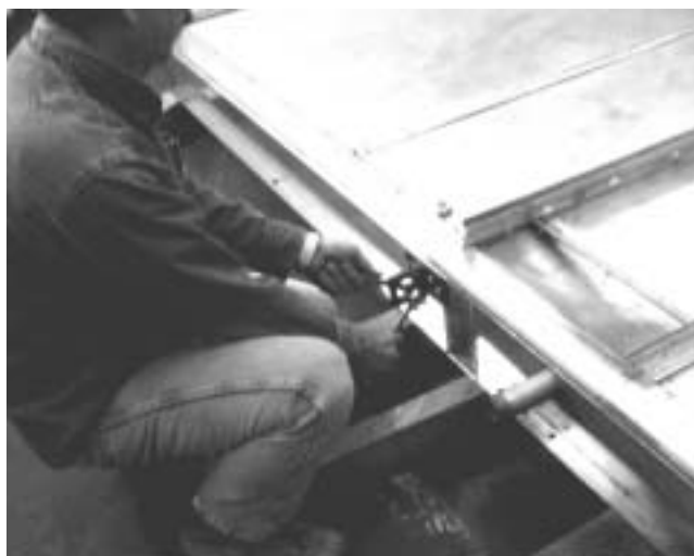
FIG. 24 - REMOVE HARDWARE AT LIFTING LUG
