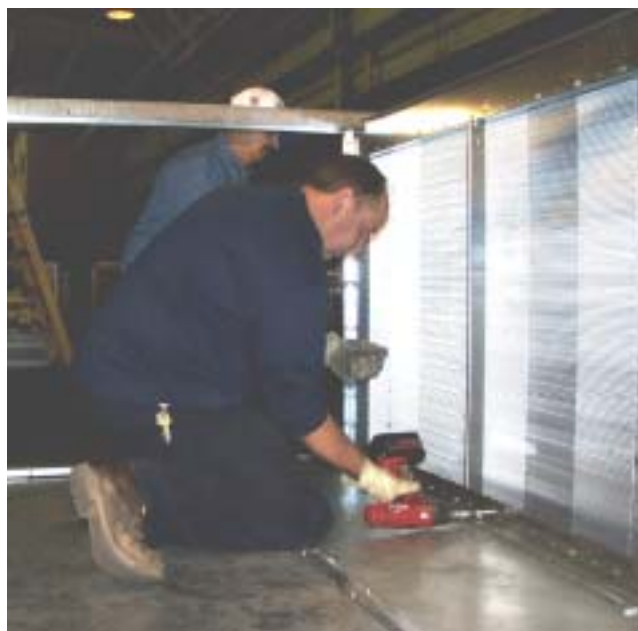
FIG. 18 - REMOVE SCREWS SECURING COIL
