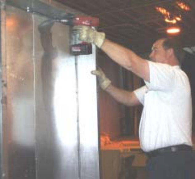
FIG. 27 - REMOVE SCREWS FROM BOTTOM OF FLOOR PANEL(S)
