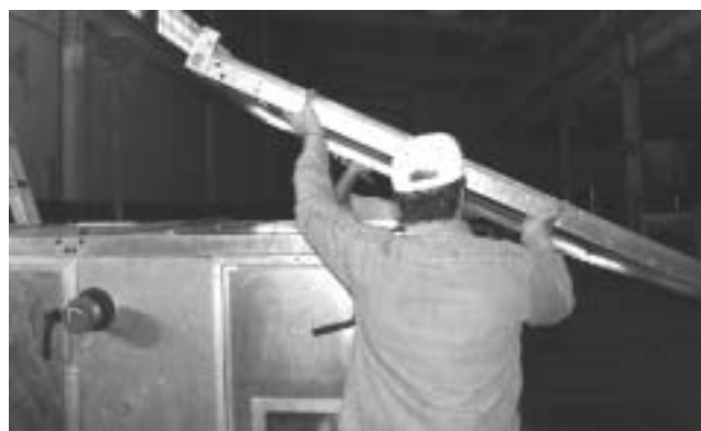
FIG. 12 - REMOVE BOTTOM RACEWAYS
