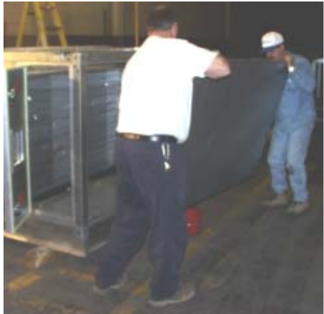
FIG. 14 - REMOVE LOWER BACK END PANEL(S)
