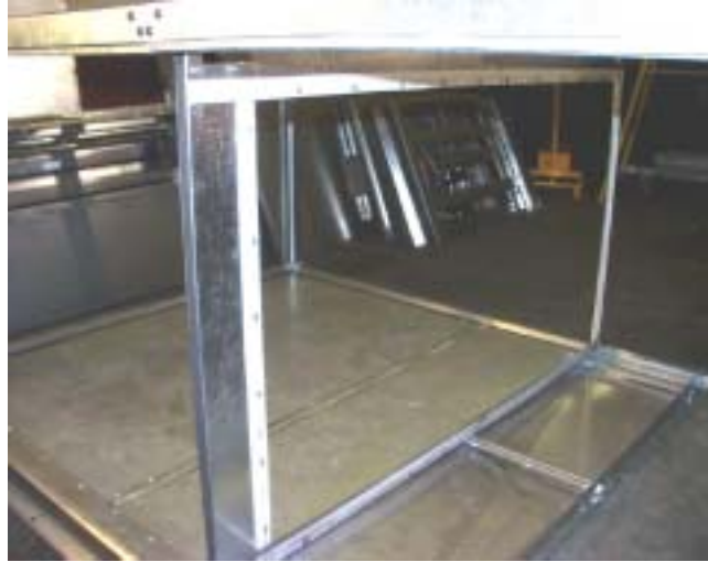
FIG. 21 - REMOVE COIL BULKHEAD
