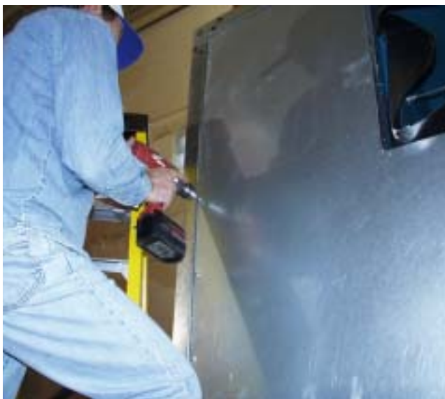
FIG. 5 - REMOVE END PANELS
