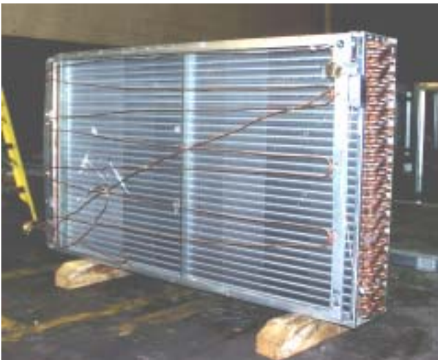
FIG. 20 - BLOCK COIL
