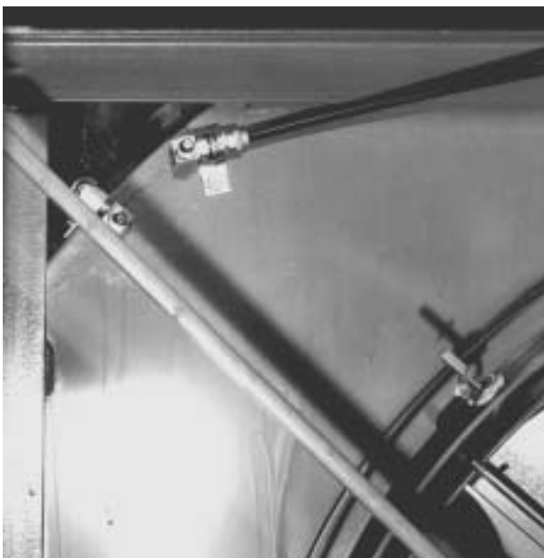
FIG. 41 – LUBRICATION LINES
