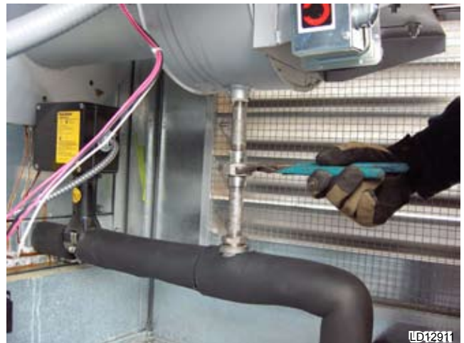
FIG. 3-19 – CONDENSATE DRAIN
