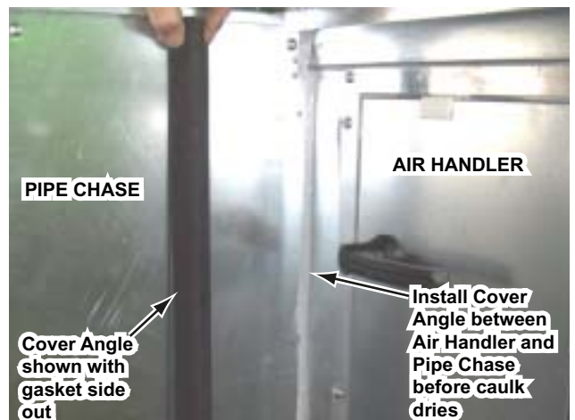
FIG. 8 – INSTALL COVER ANGLE
