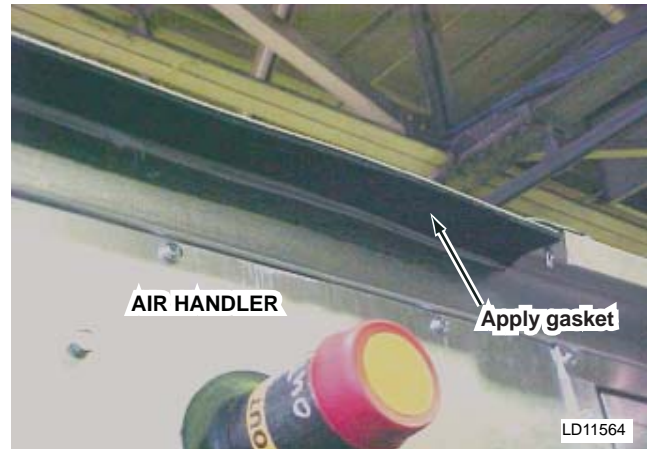
FIG. 1 – INSTALL GASKET UNDER ROOF OVERHANG
