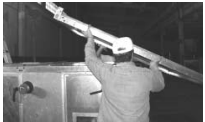
FIG. 12 - REMOVE BOTTOM RACEWAYS
