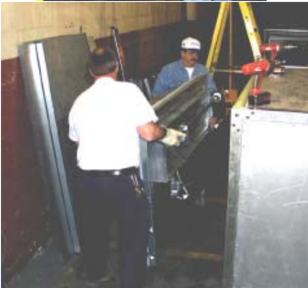
FIG. 13 - REMOVE BOTTOM FRONT END PANEL(S)
