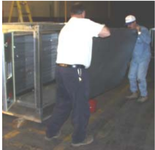
FIG. 14 - REMOVE LOWER BACK END PANEL(S)
