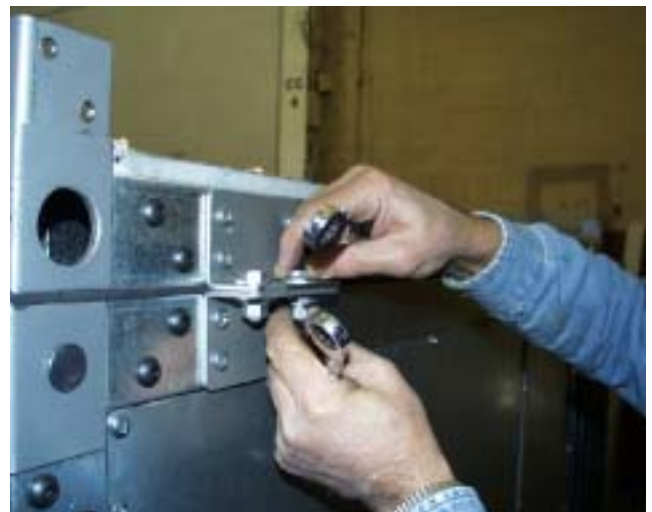
FIG. 11 - REMOVE HARDWARE FROM TOP SECTION MOUNTING BRACKETS
