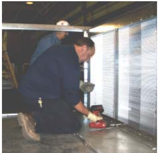
FIG. 18 - REMOVE SCREWS SECURING COIL
