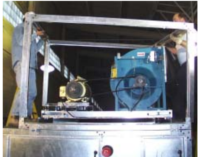
FIG. 7 - REMOVE TOP RACEWAY ASSEMBLY
