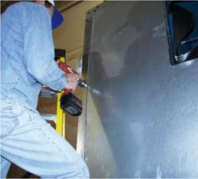
FIG. 5 - REMOVE END PANELS
