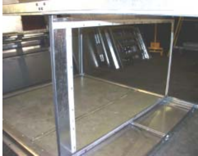
FIG. 21 - REMOVE COIL BULKHEAD
