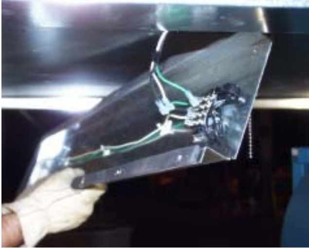
FIG. 16 - REMOVE ELECTRICAL CONNECTORS
