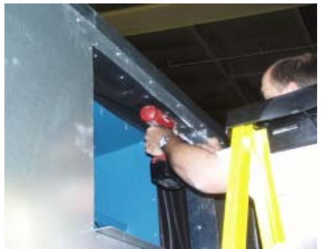
FIG. 4 - DISCONNECT FAN DISCHARGE FLEX CONNECTOR
