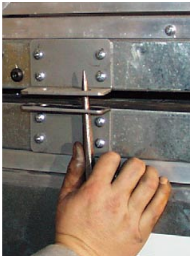
FIG. 2-18 – GUIDING BRACKETS TOGETHER
