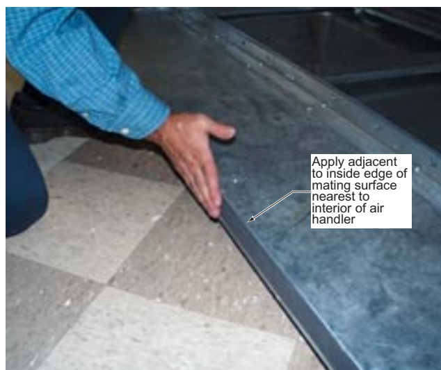
FIG. 2-9 – APPLYING GASKET
