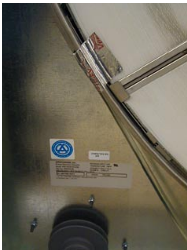
FIG. 5-46 – ATTACHING THE HOOK END OF BELT TO WHEEL RIM WITH TAPE
