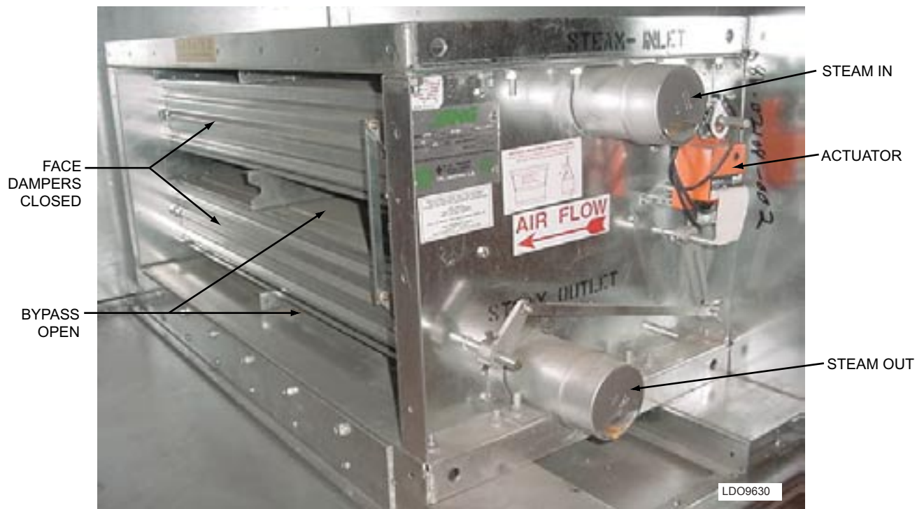
FIG. 2-25 – INTEGRAL FACE & BYPASS COIL (HORIZONTAL; TUBES, STEAM SHOWN)
