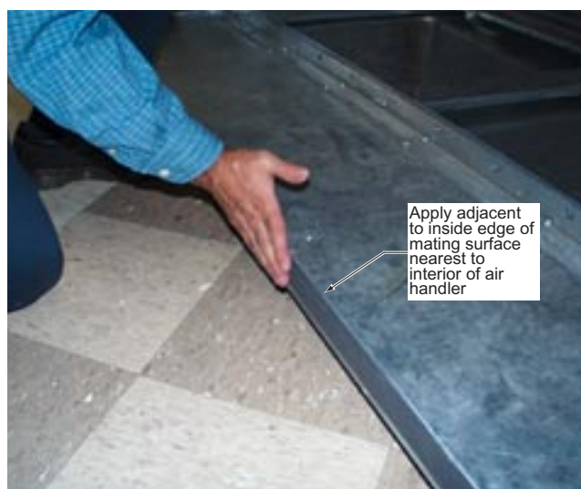
FIG. 2-17 – APPLYING GASKET
