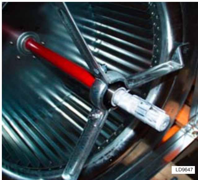
FIG. 4-6 – SEALED BEARING
