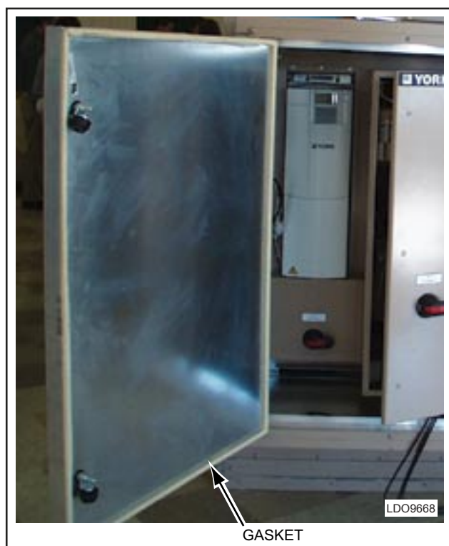
FIG. 5-26 – REPLACEMENT OF DOOR GASKET
