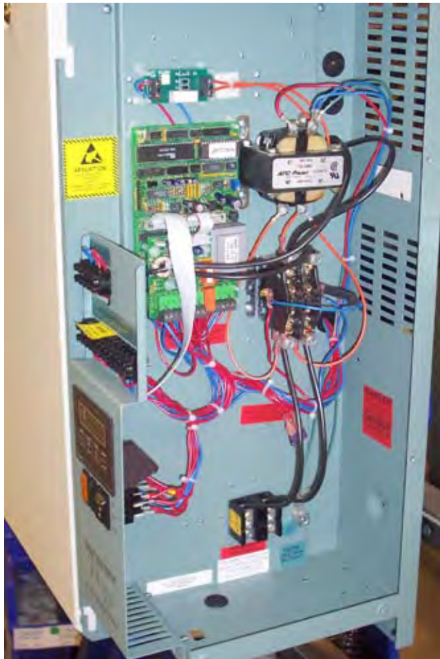
FIG. 2-62 – TYPICAL HUMIDIFIER PANEL LAYOUT
