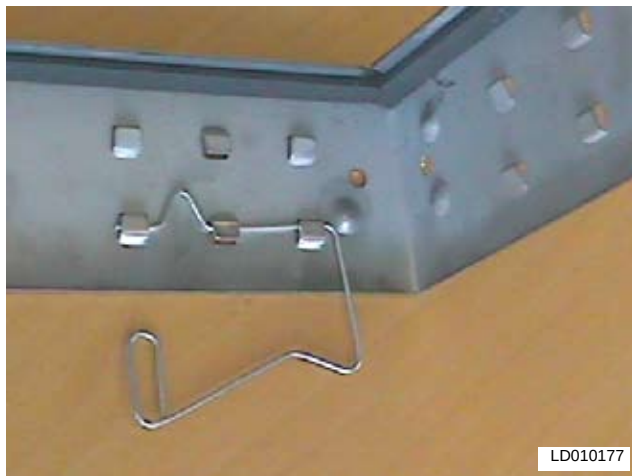
FIG. 2-101 – CORRECTLY INSTALLED LATCH P/N 026-35778-007
