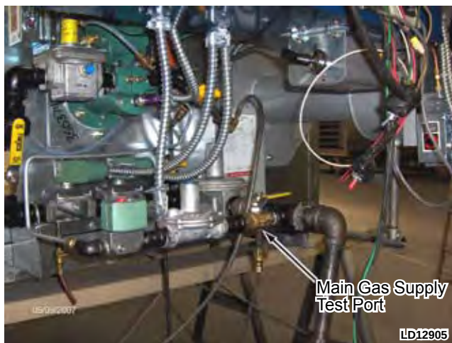
FIG. 3-16 – CHECK MAIN GAS SUPPLY PRESSURE
