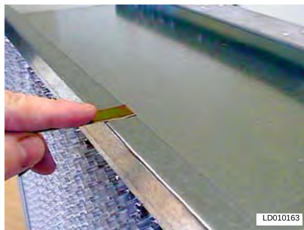
FIG. 2-112 – PREFILTER LATCH AFTER INSTALLATION ONTO FILTER HEADER.
