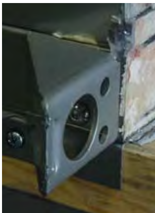
Raceway Lifting Lug (at shipping split)
