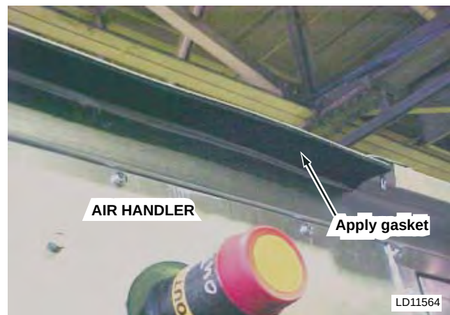
FIG. 2-41 – INSTALL GASKET UNDER ROOF OVERHANG
