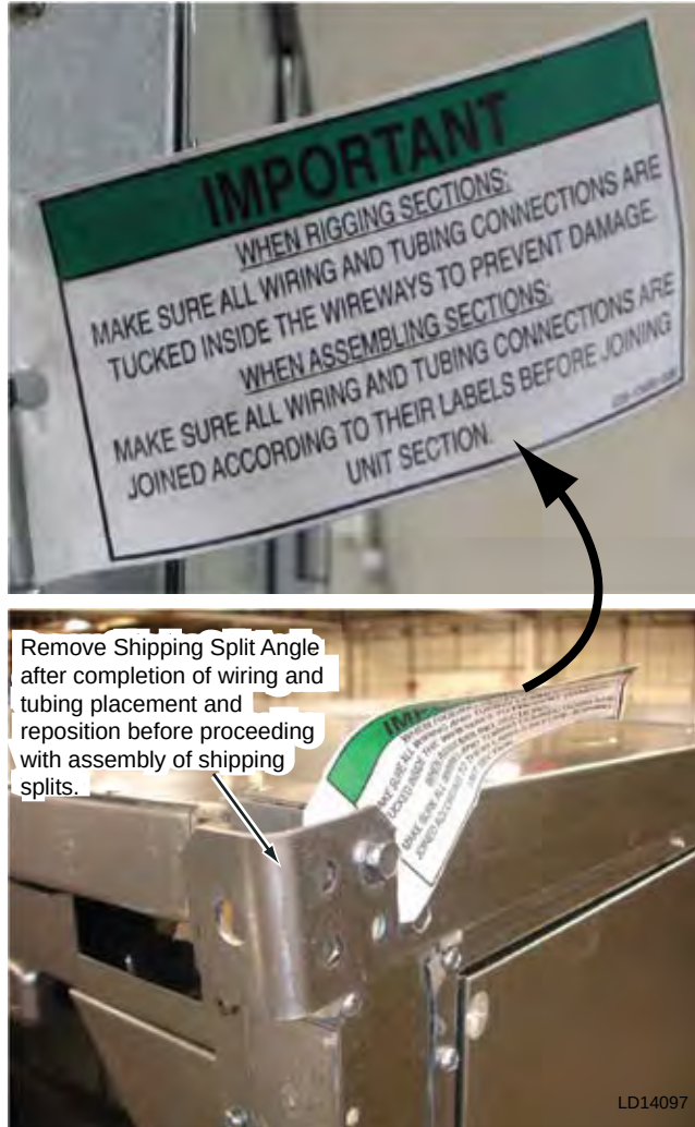
FIG. 2-19 – REMOVE AND REPOSITION SHIPPING SPLIT ANGLE
