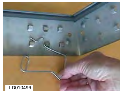
FIG. 2-104 – INSTALL LATCH P//N 026-35778-007
