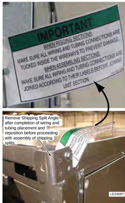
FIG. 2-24 – REMOVE AND REPOSITION SHIPPING SPLIT ANGLE
