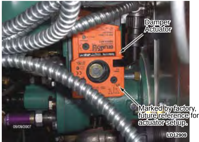
FIG. 3-19 – DAMPER ACTUATOR
