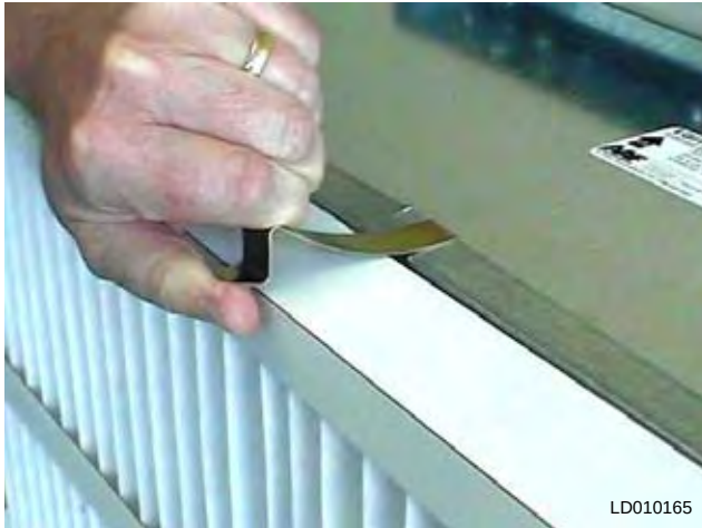
FIG. 2-113 – POSITION PREFILTER IN FRONT OF THE FINAL FILTER. (2" W/026-36339-000 LATCH SHOWN)
