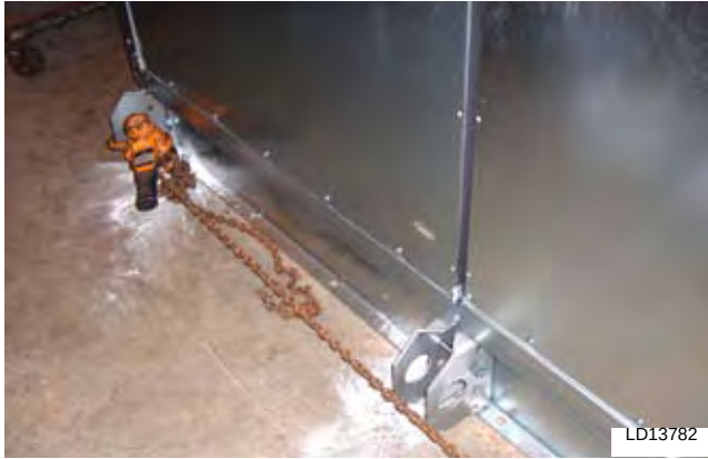
FIG. 2-25 – PLACING AND ANCHORING FIRST SECTION AND ATTACHING COME-A-LONGS
