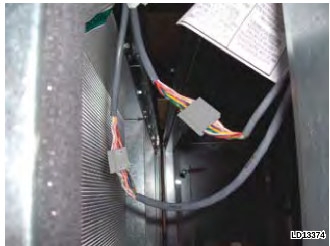
FIG. 2-27 – ELECTRICAL CONNECTIONS
