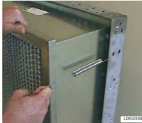
FIG. 2-111 – FRAME WITH 4 LATCHES INSTALLED
