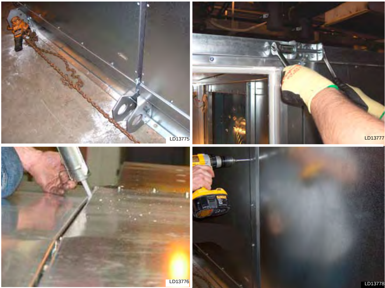
FIG. 2-20 – BRINGING SECTIONS TOGETHER
