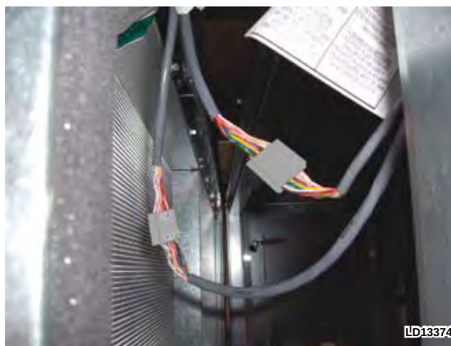
FIG. 2-18 – ELECTRICAL CONNECTIONS
