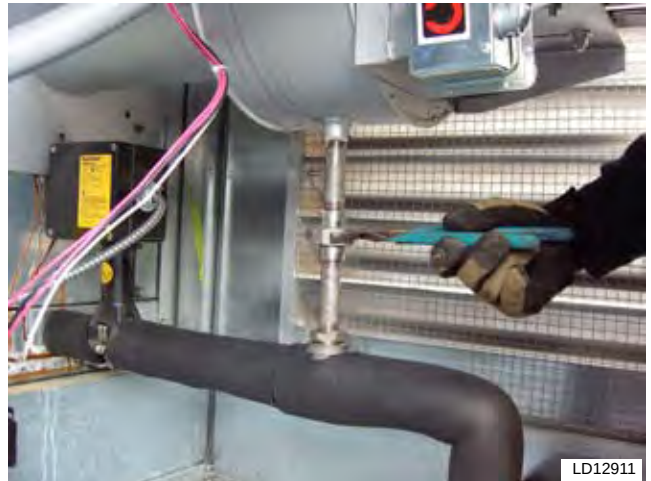
FIG. 3-20 – CONDENSATE DRAIN
