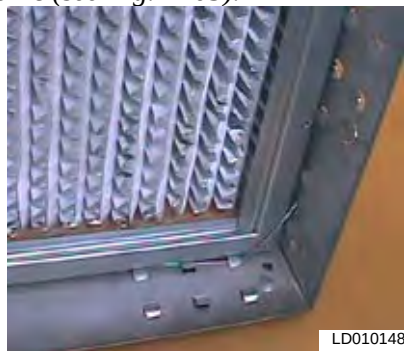
FIG. 2-103 – INSTALLED CARTRIDGE FILTER
