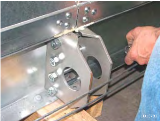
FIG. 2-28 – INSTALLING BOLTS AFTER PULLING UNITS TIGHT TOGETHER
