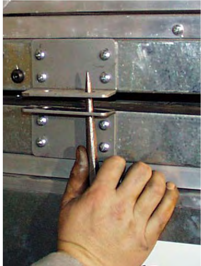
FIG. 2-32 – GUIDING BRACKETS TOGETHER
