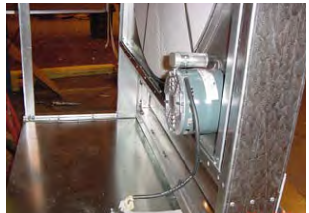
FIG. 2-55 – TYPICAL POWER WIRING OF ENERGY RECOVERY WHEEL
