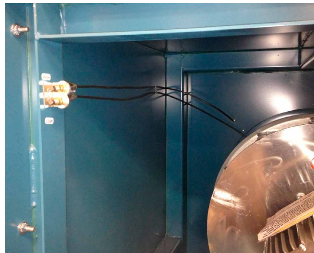
FIGURE 83 - HIGH AND LOW CONNECTIONS AND ASSOCIATED TUBING FOR FAN MOUNTED AIR MONITORING SYSTEM
