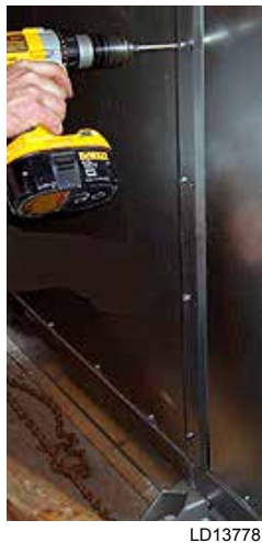
FIGURE 63 - INSTALLING GASKETS
