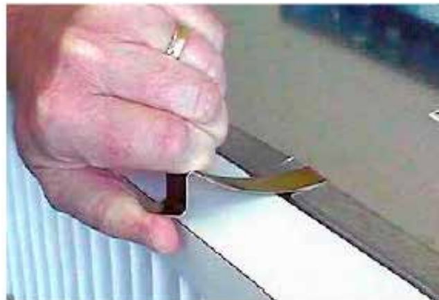
FIGURE 162 - POSITION PRE-FILTER IN FRONT OF FINAL FILTER
