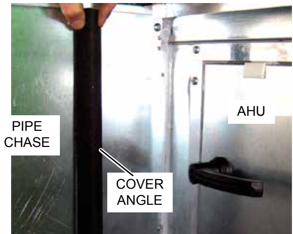
FIGURE 92 - INSTALL COVER ANGLE
