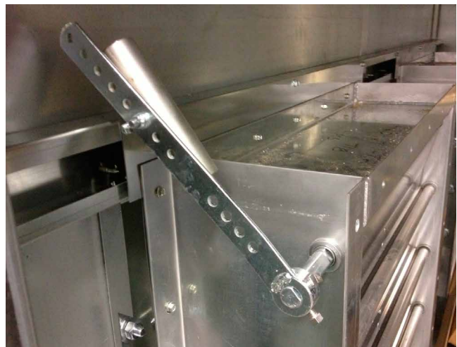
FIGURE 76 - COUNTERBALANCE UNLOCKED FOR START-UP
