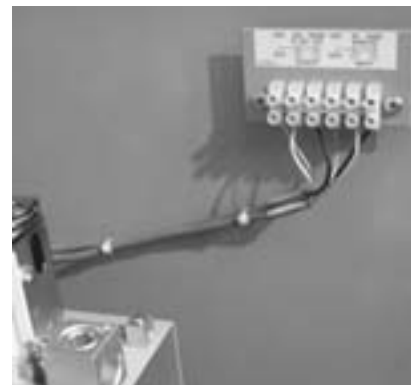
TYPICAL FIELD TERMINATIONS
