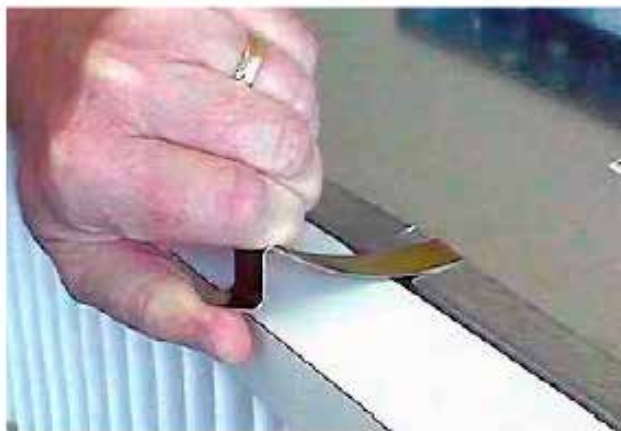
FIGURE 48 - POSITION PREFILTER IN FRONT OF THE FINAL FILTER (2" W/026-35788-625 LATCH SHOWN)
