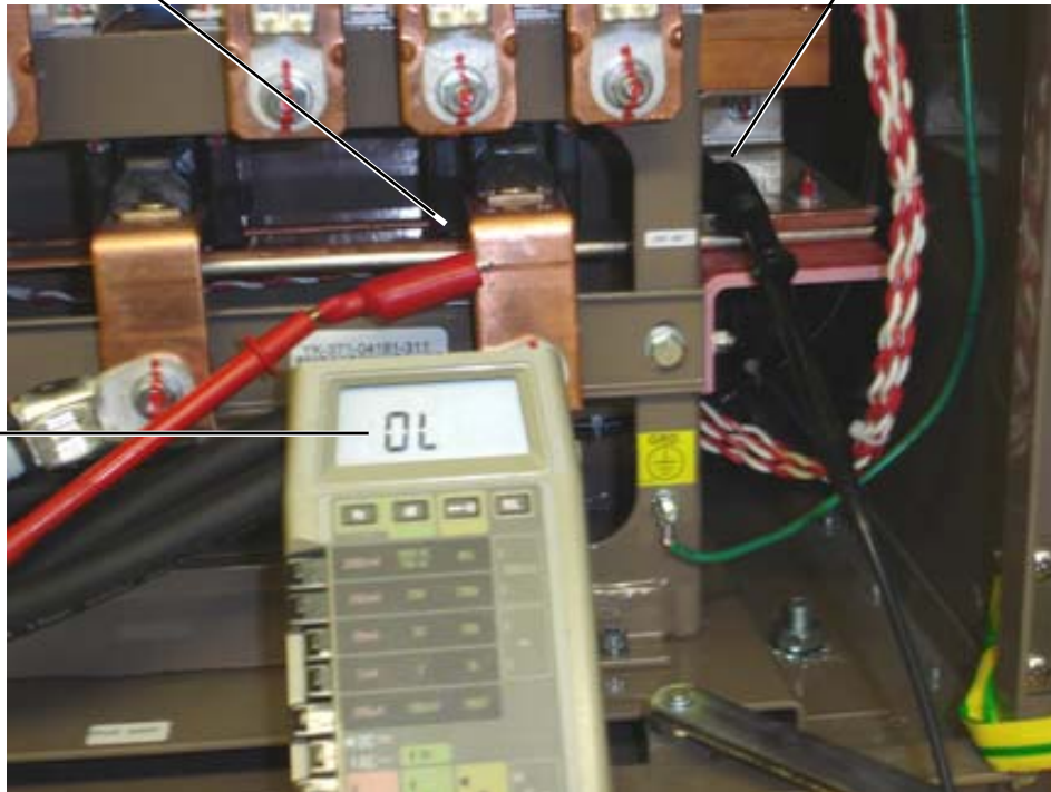
FIG. 10 – SCR / DIODE MODULE VERIFICATION #2
