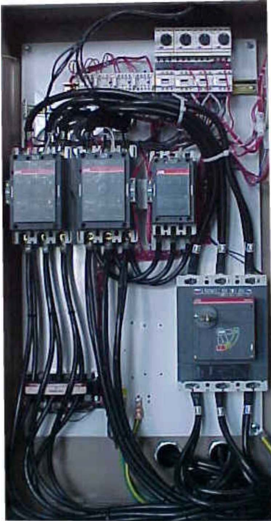
FIG. 12 – WYE DELTA POWER PANEL
