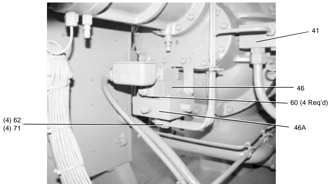
FIG. 8 – 4-WAY SOLENOID VALVE AND SUBPLATE
