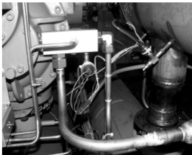
FIG. 18 – OIL PRESSURE TRANSDUCER LOCATION
