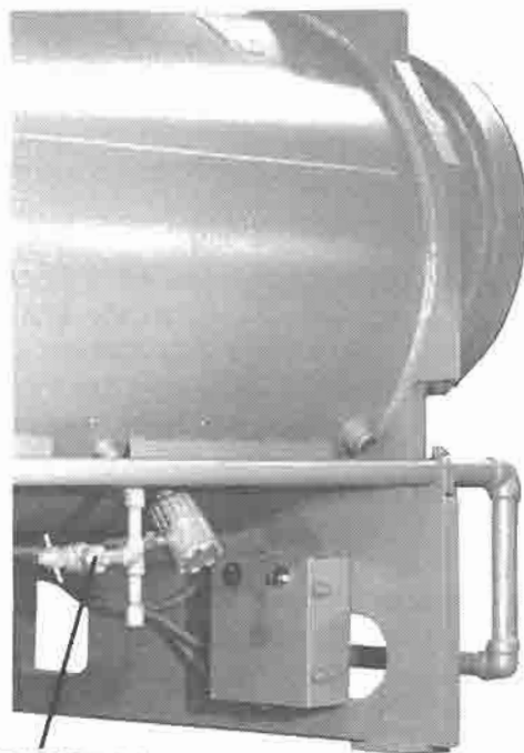
REFRIGERANT & EVACUATION CHARGING VALVE
