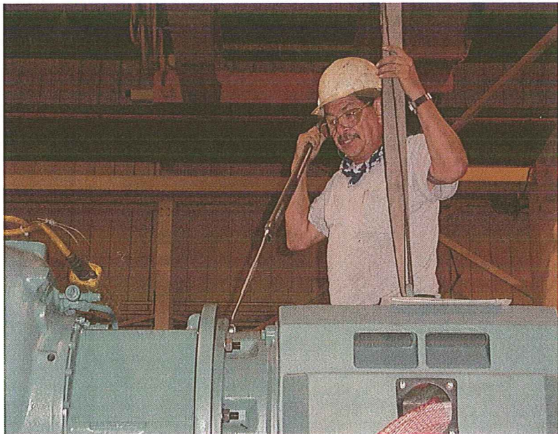
Tighten motor to compressor.
