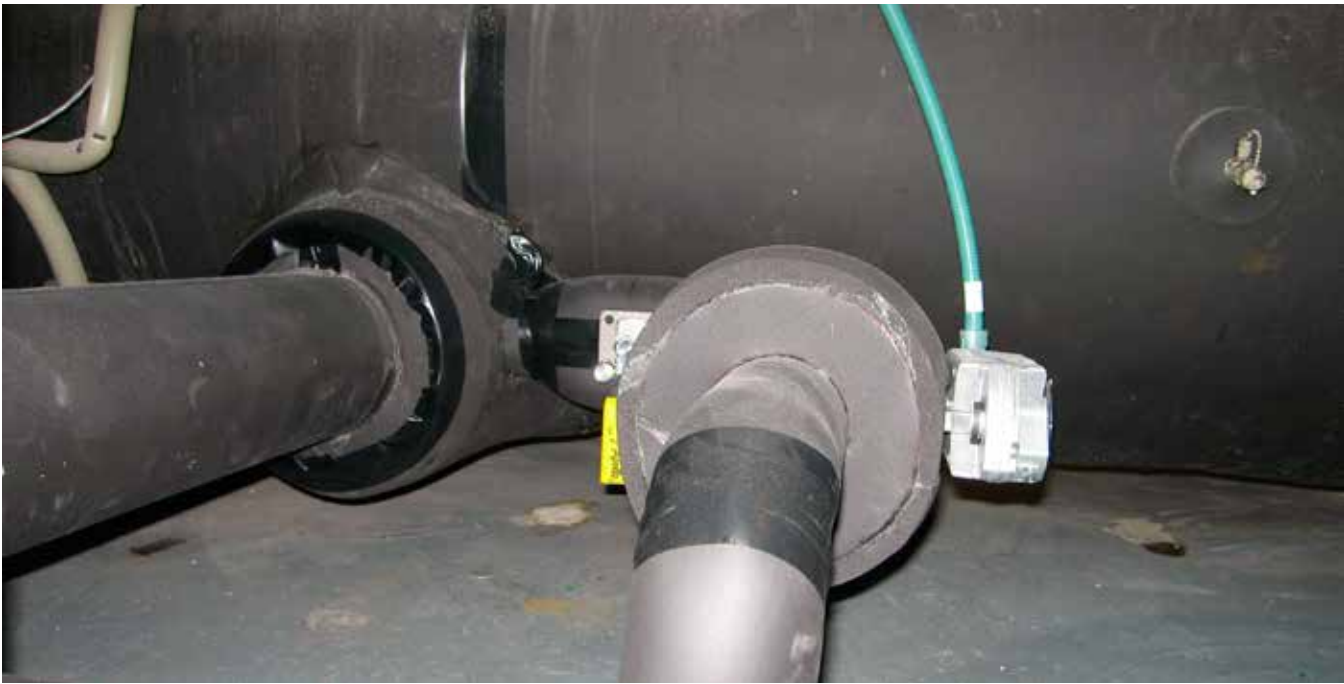
FIGURE 71 - LIQUID/ORIFICE BYPASS EXAMPLE
