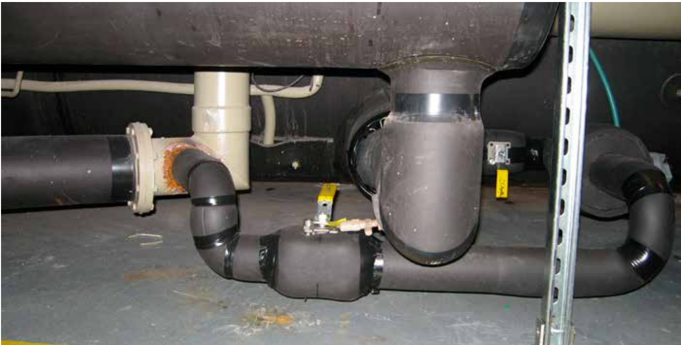
FIGURE 72 - LIQUID/ORIFICE BYPASS EXAMPLE
