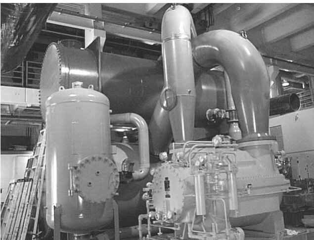
FIG. 14 - MAJOR REFRIGERANT PIPING ASSEMBLY
