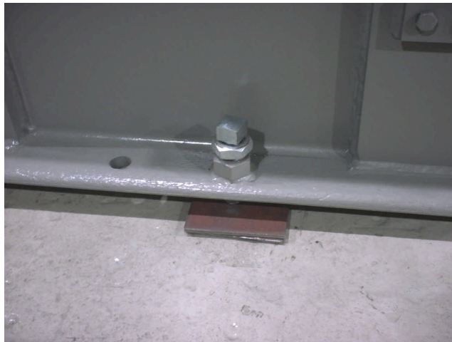
Steel plates under jackbolts to prevent gouging pad.
